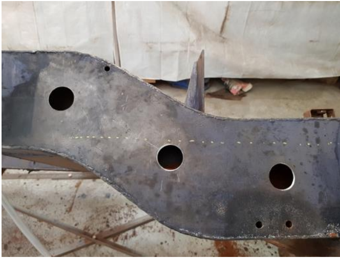
Dirt Removal Holes #1
