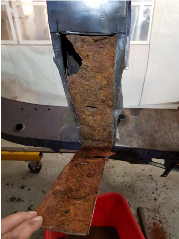
Dirt in Crossmember
