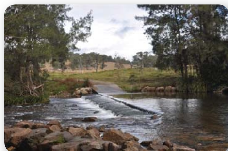
Water Crossing NE of Gloucester
